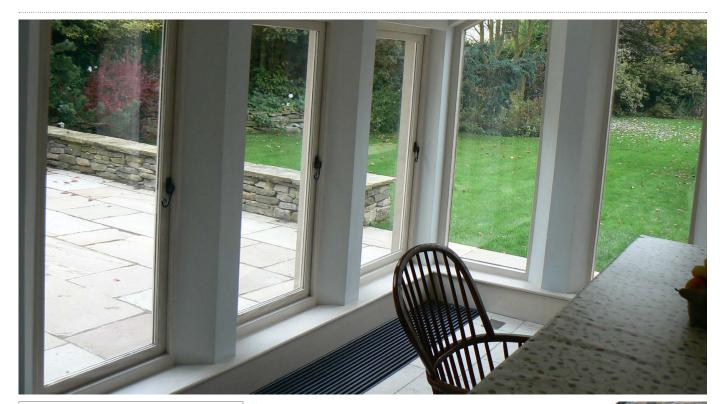
"Due to the home being a Grade II listed dwelling in the Peak District National Park, the extension was challenging. Radiators were ruled out due to the lack of wall space. The MEINERTZ ProLine provided a faster warm up time than underfloor heating, whilst providing a heat source in front of the colder windows."
